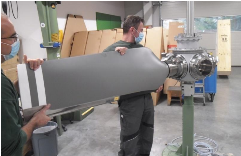
Figure 8: Installation of the blade only with two mechanics
