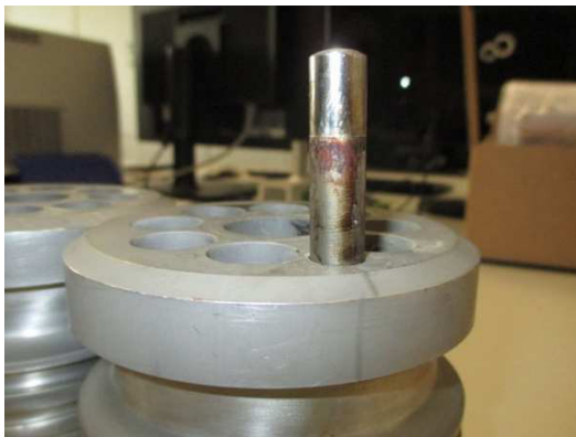
Figure 3: Corrosion on pitch change pin
