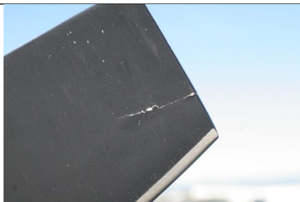
Split Blade tip. Repair with fiber glass
