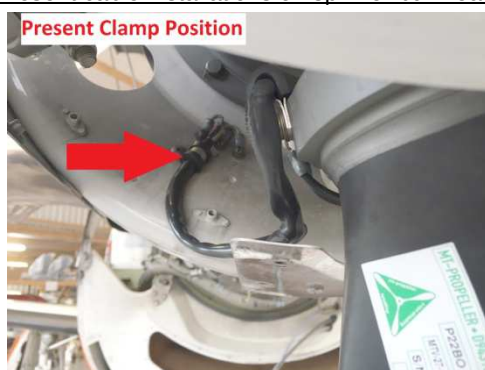
Present cable installations on spinner bulkhead
