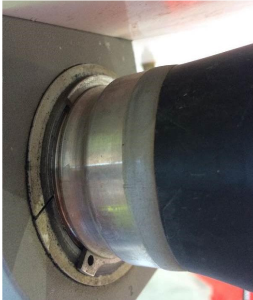
Figure 1: Example of damaged snap ring still in place
